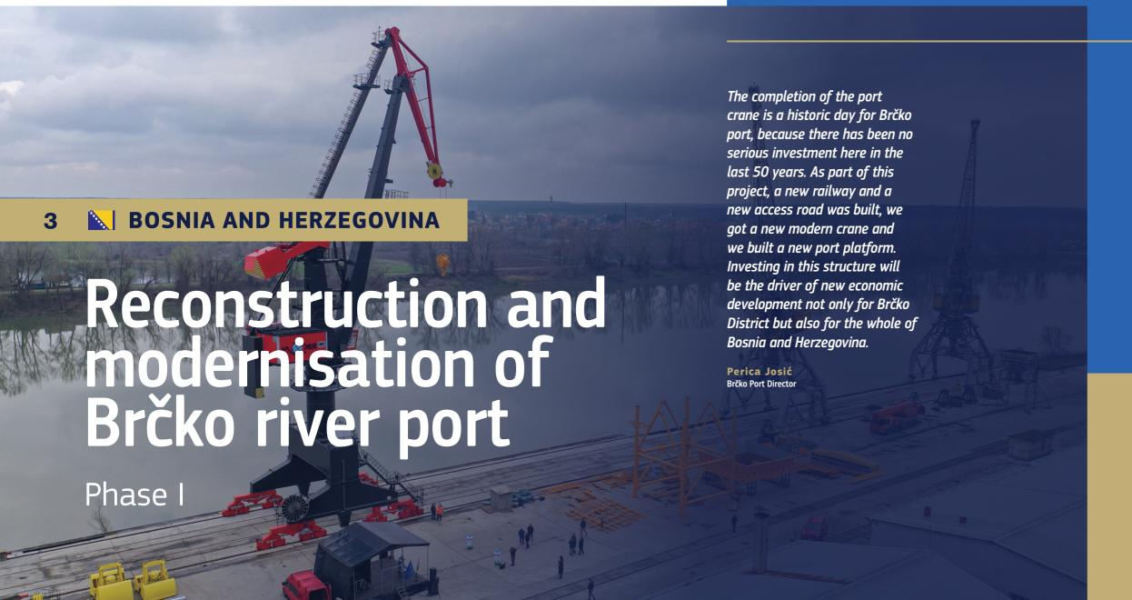
This project includes the construction and arrangement of the port plateau, the purchase of a new crane, the reconstruction of the access road from the port to Bijeljinska Cesta as well as the industrial railway from the port to Brčko Novo railway station. The new crane triples the capability of the previous one. This improvement is expected to significantly increase the port's efficiency.
