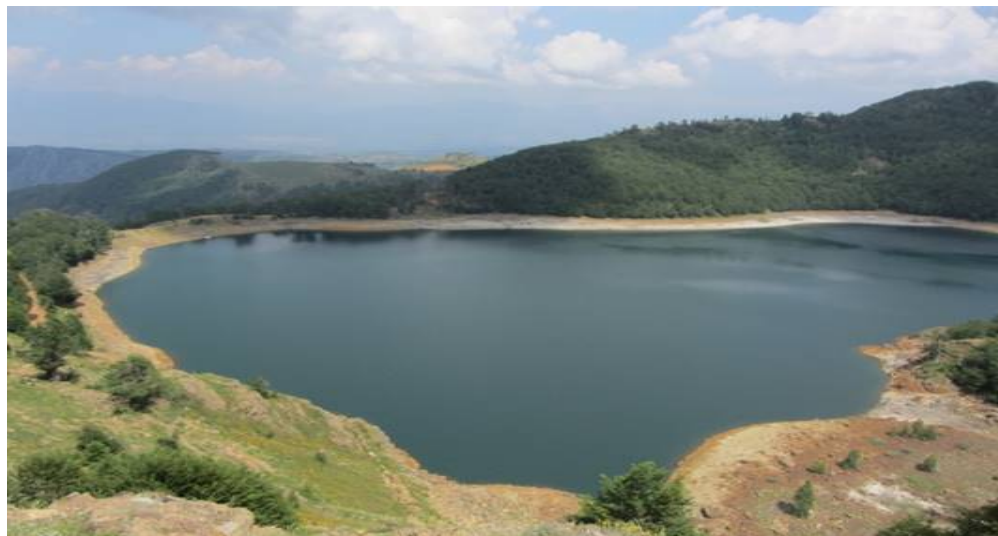
Ternoves Hydropower Plant, Albania
