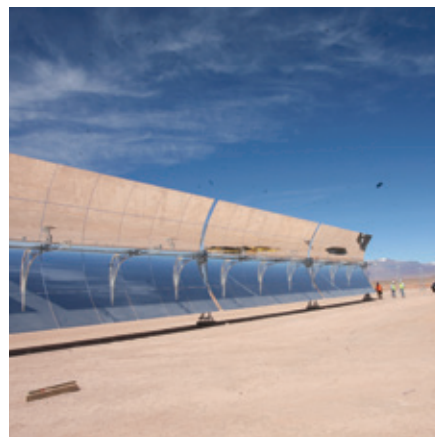
Ouarzazate Solar Plant. ©EIB Photo Library
